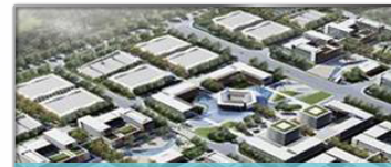
Operator M, Smart DCIM, Improve Management Efficiency by 50%
